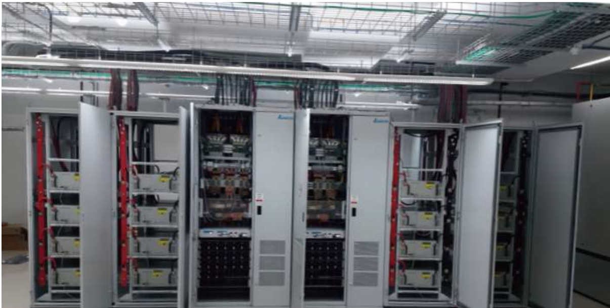
India Reliance Data Center Project
